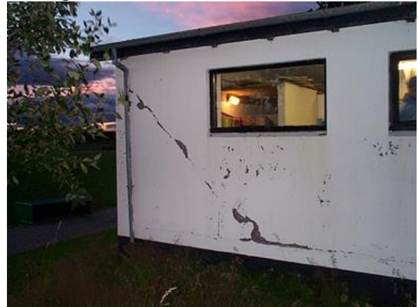
Figure 6: Damaged squat wall in Hveragerði after the 2000 earthquake with visible shear crack.
